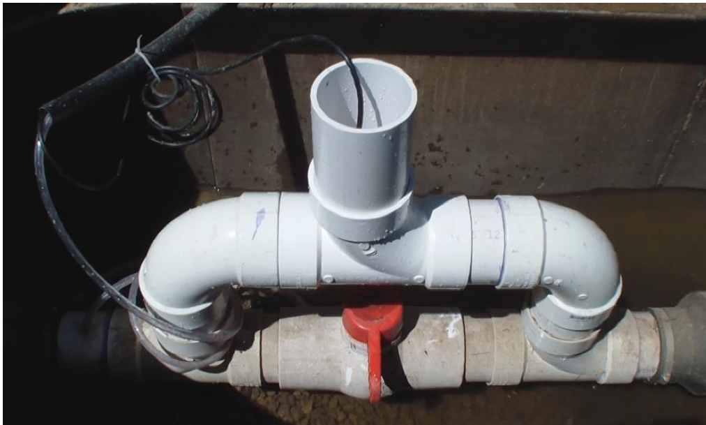
Figure 2: The underdrain riser installed in 2014 to encourage infiltration.
