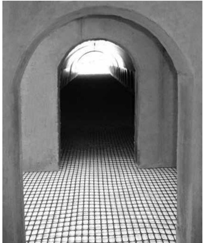
A distribution manifold is typically located at one end of every row of arches. Inspection can be done through manhole access and visually inspecting the distribution manifold. When the depth of sediment accumulates over 4 inches (102 mm), cleanout is recommended.
